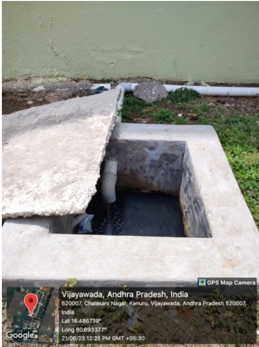
Liquid Waste Generated diverted into Soak Pits
